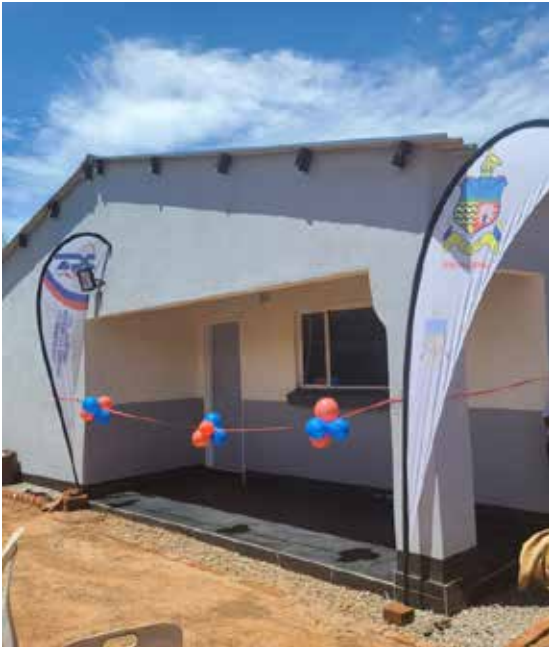
The newly constructed house for Chief Deli reflects ZESA's commitment to community development and sustainable empowerment.
